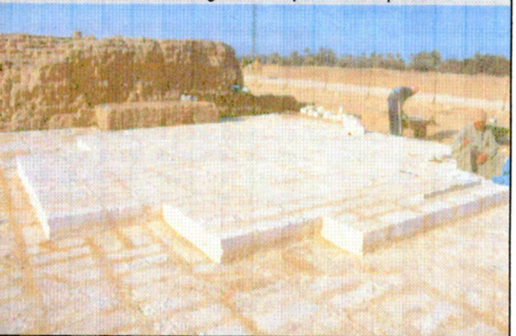
Small Aten Temple. Central gateway at the 1st pylon. Replacing the original stone pavement & platform.
