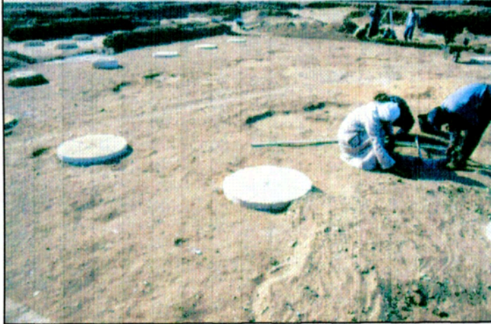
North Palace. Central Hall: preparing new cement pad for new column base.
